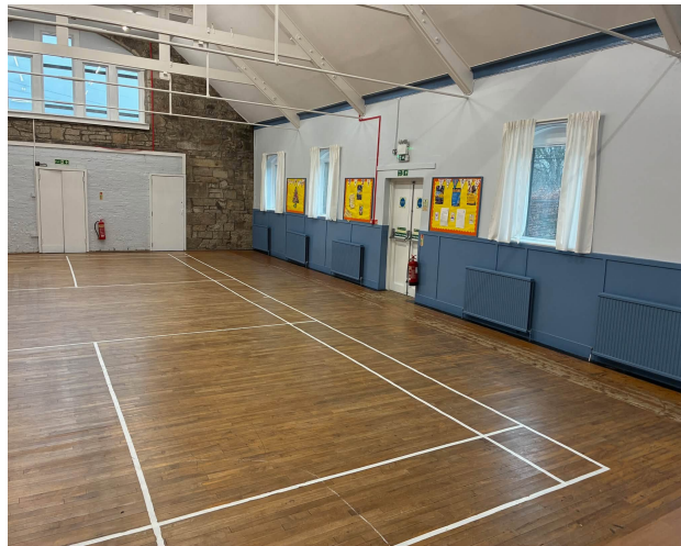
A view of the Main Hall prior to commencement of radiator replacement
